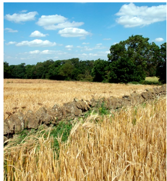
Drystone Walling and Footpath, Ketton
